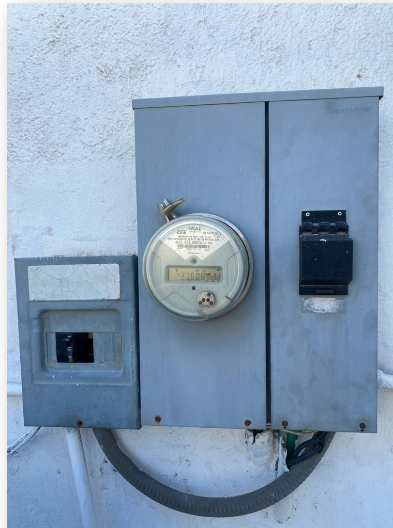
Medidor CFE controla caseta y portones / CFE meter controls guardhouse and gates
