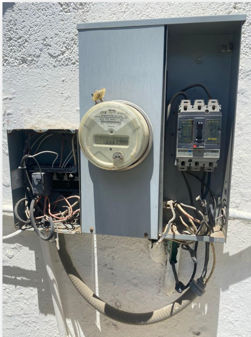
Medidor CFE controla caseta y portones / CFE meter controls guardhouse and gates
